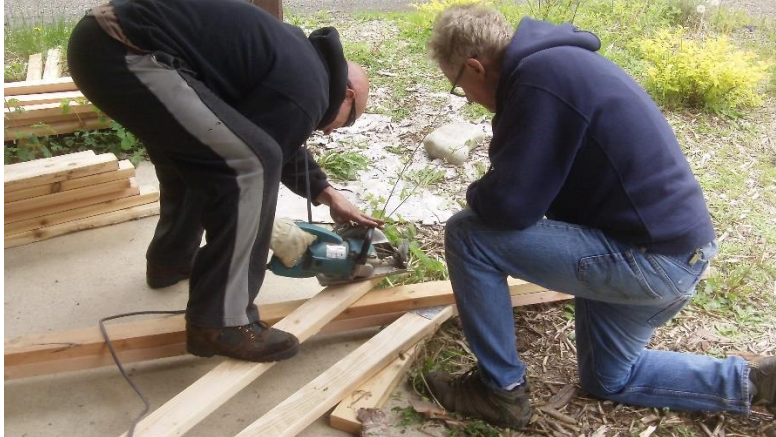
Here John Schindler is sawing cross braces for the second truss.
